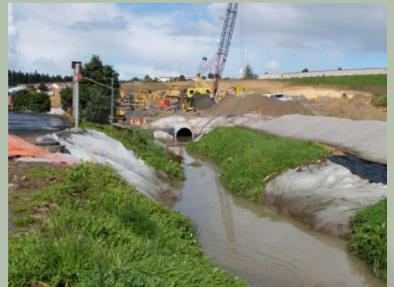
An Oakley Creek tributary is being put into a 372 m long culvert at the Maoro Rd Interchange on SH20 behind the Stoddard Rd shops - and there's much more of this type of work to come (see left). There were 145 short fin eels captured from here and released downstream into Oakley Creek at Alan Wood Reserve. Was there any research to determine the impact of this translocation? What other fauna and flora was left behind or destroyed? The high sediment load which can be seen in the photo was attributed by NZTA contractors to other housing developments upstream.
